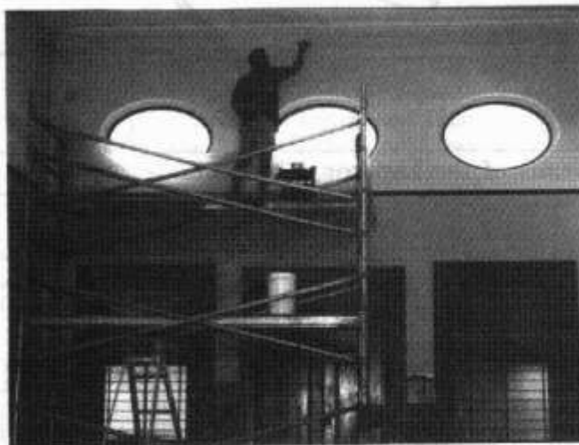
The Instrument Room during restoration. By Glen Blaxland.
