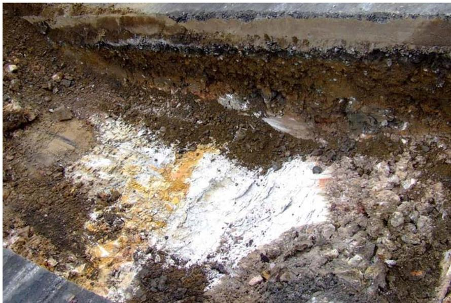
Figure 4 A weathered igneous dyke in a trench
